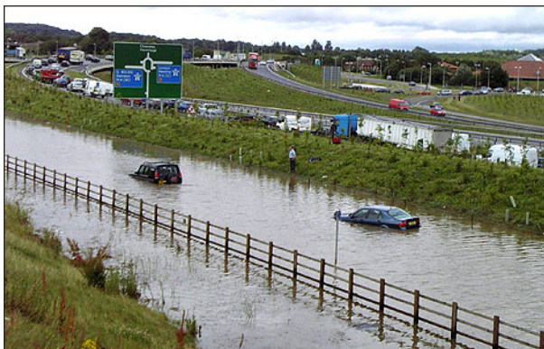
A34 Chieveley south of M4 Junction 13
